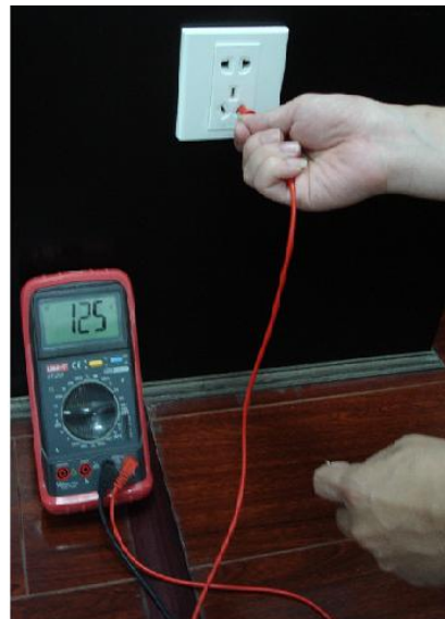
Appendix Figure 7-6 Check live cable connection
