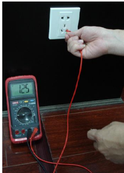
Appendix Figure 7-6 Check live cable connection
